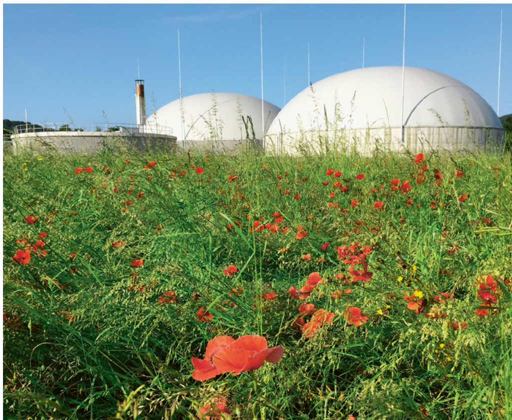
Our Henniez bottled-water plant in Switzerland produces renewable energy by collecting and burning manure from local cattle in a biogas plant, together with spent coffee grounds from Nespresso .
